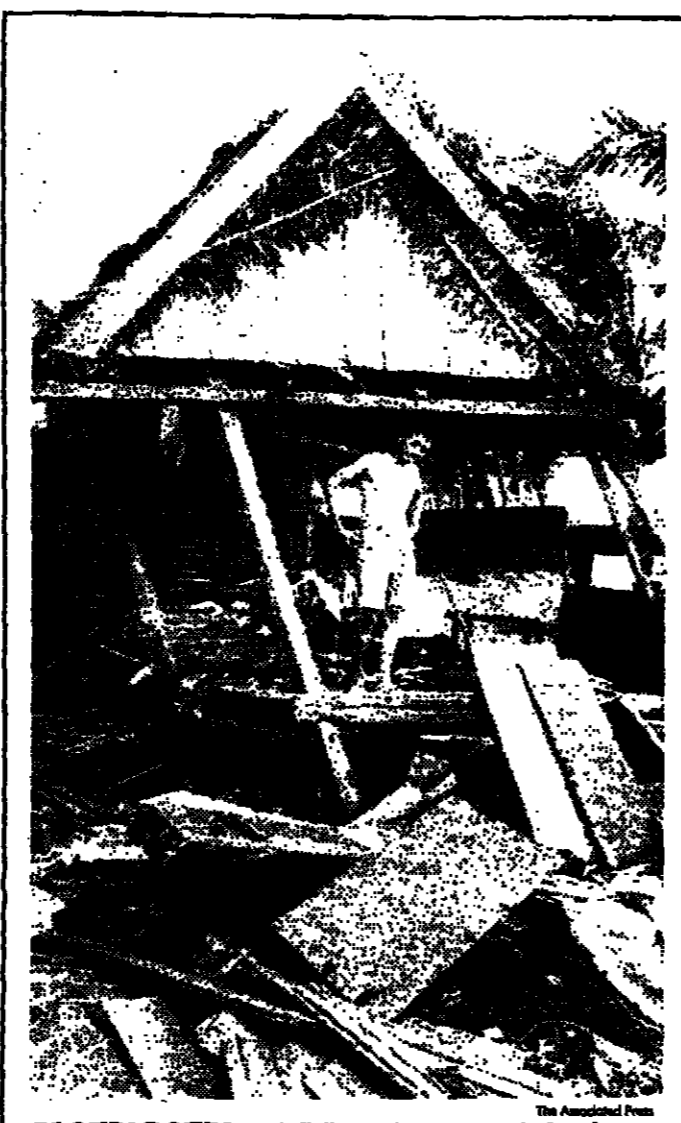
BLOWN DOWN — A Filipino farmer stands in what remained of his house after a typhoon, designated Irma, swept across the southeastern Philippines this week. Waves generated by the storm smashed a coastal town in Cansines province, killing 136 of the 158 recorded fatalities.
